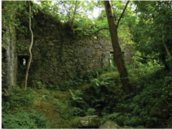
Figure 4 - Ellan Vhow Castle Interior (south). "Dungeon" entrance is just past the mature tree (right center).
